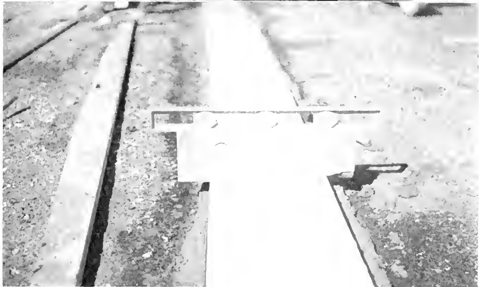
UPPER—Spreading mortar for curb section. LOWER—Leveling device for truing up curb.
